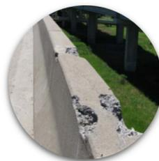
**Spalls** are a depression in a concrete caused by deterioration or removal of a portion of the concrete surface.
