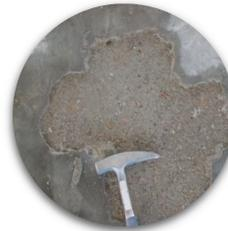
**Delamination** occurs when layers of concrete separate at or near the outermost layer of reinforcing steel, often because of deterioration of the reinforcing steel.
