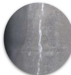
**Efflorescence** is a common term used in structure inspections and refers to the white, powdery substance left behind from water seepage or leaking that indicates concrete deterioration or cracking.
